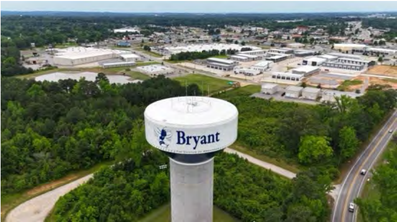
Bryant Water Tower, Hwy 5, South View
