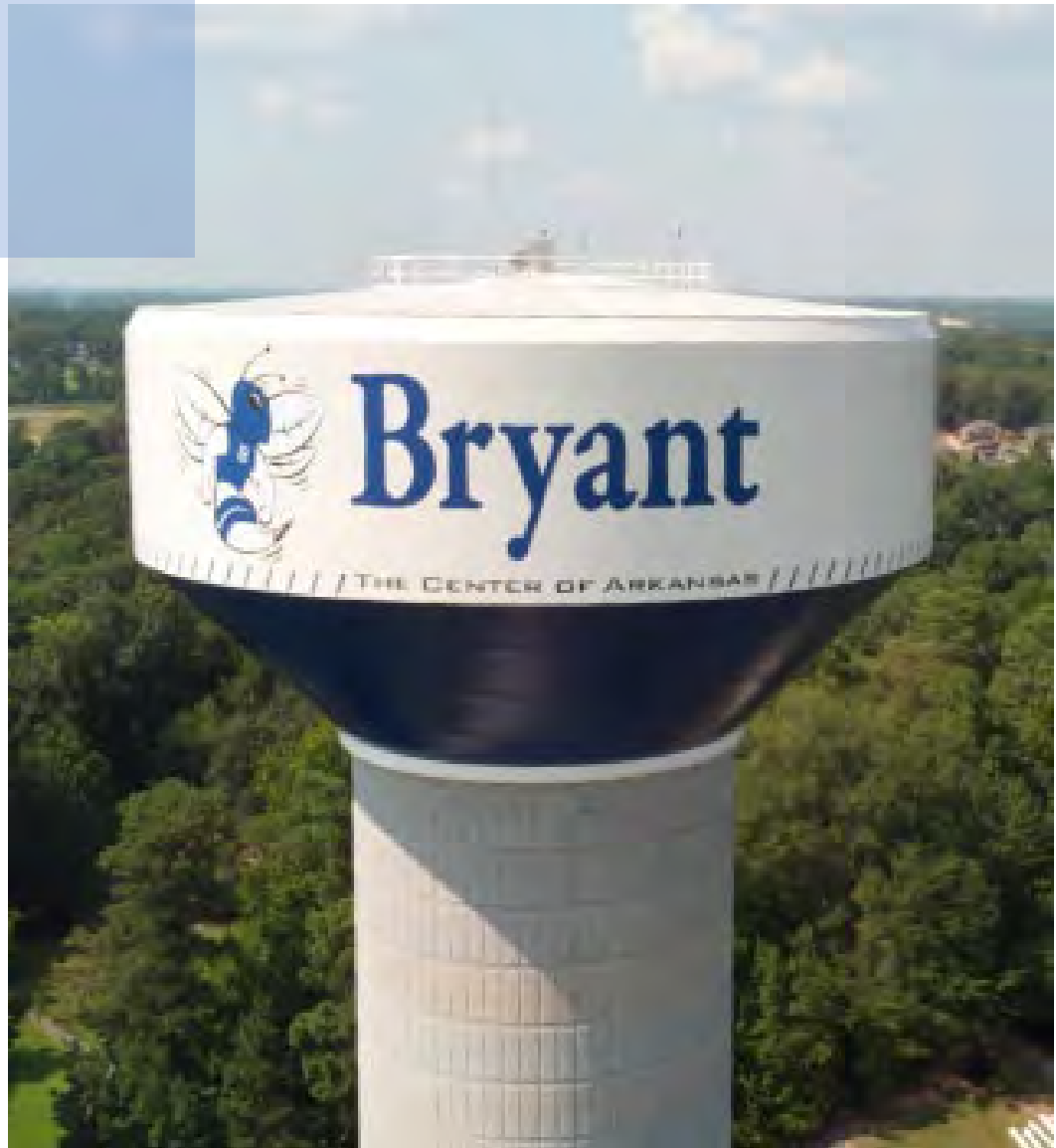
Bryant Water Tower, Hwy 5
