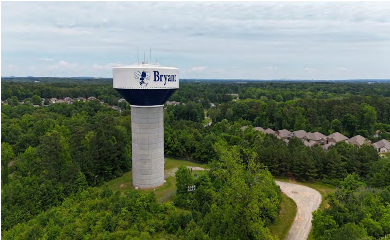
Water Tower, Hwy 5, North View
