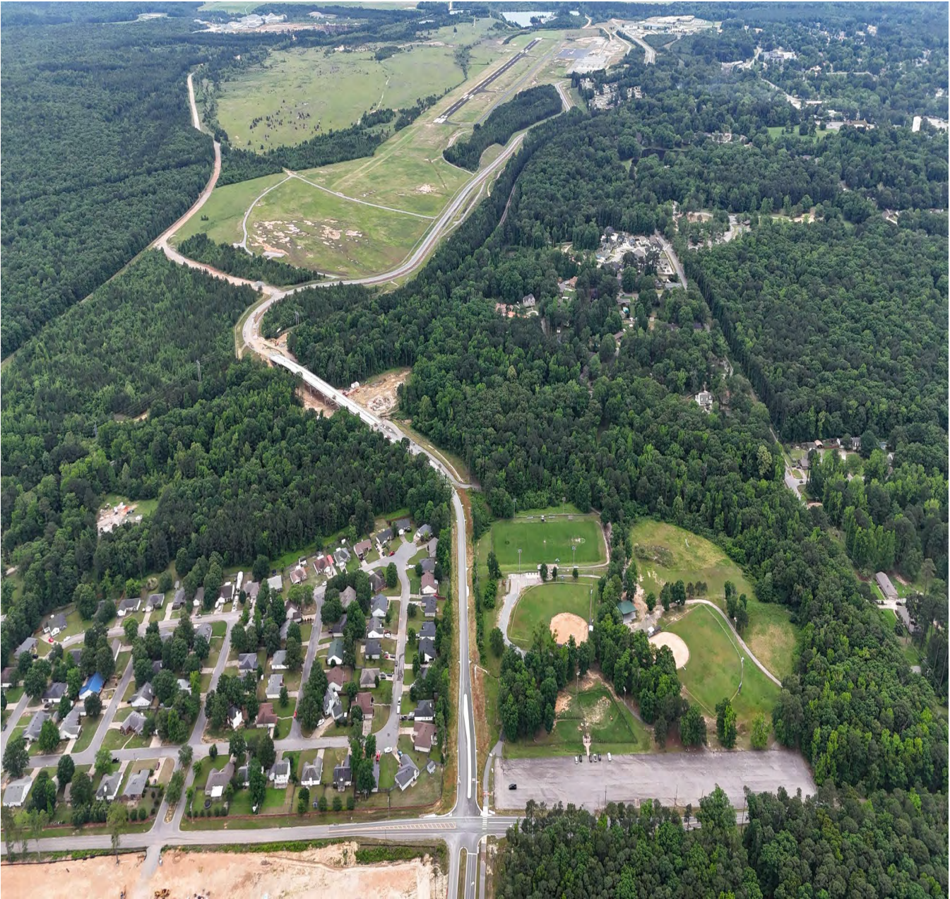
2023 Work in Progress - Bryant Parkway Phase II
