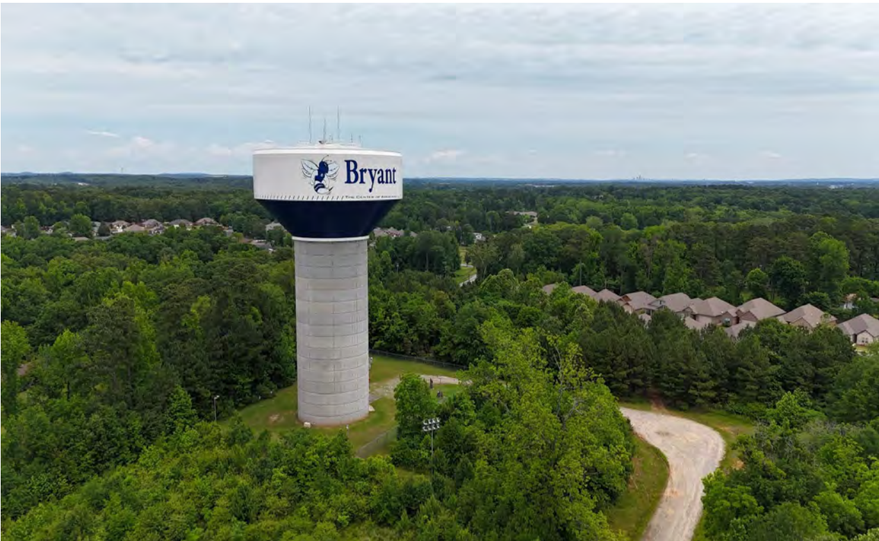
Water Tower, Hwy 5, North View
