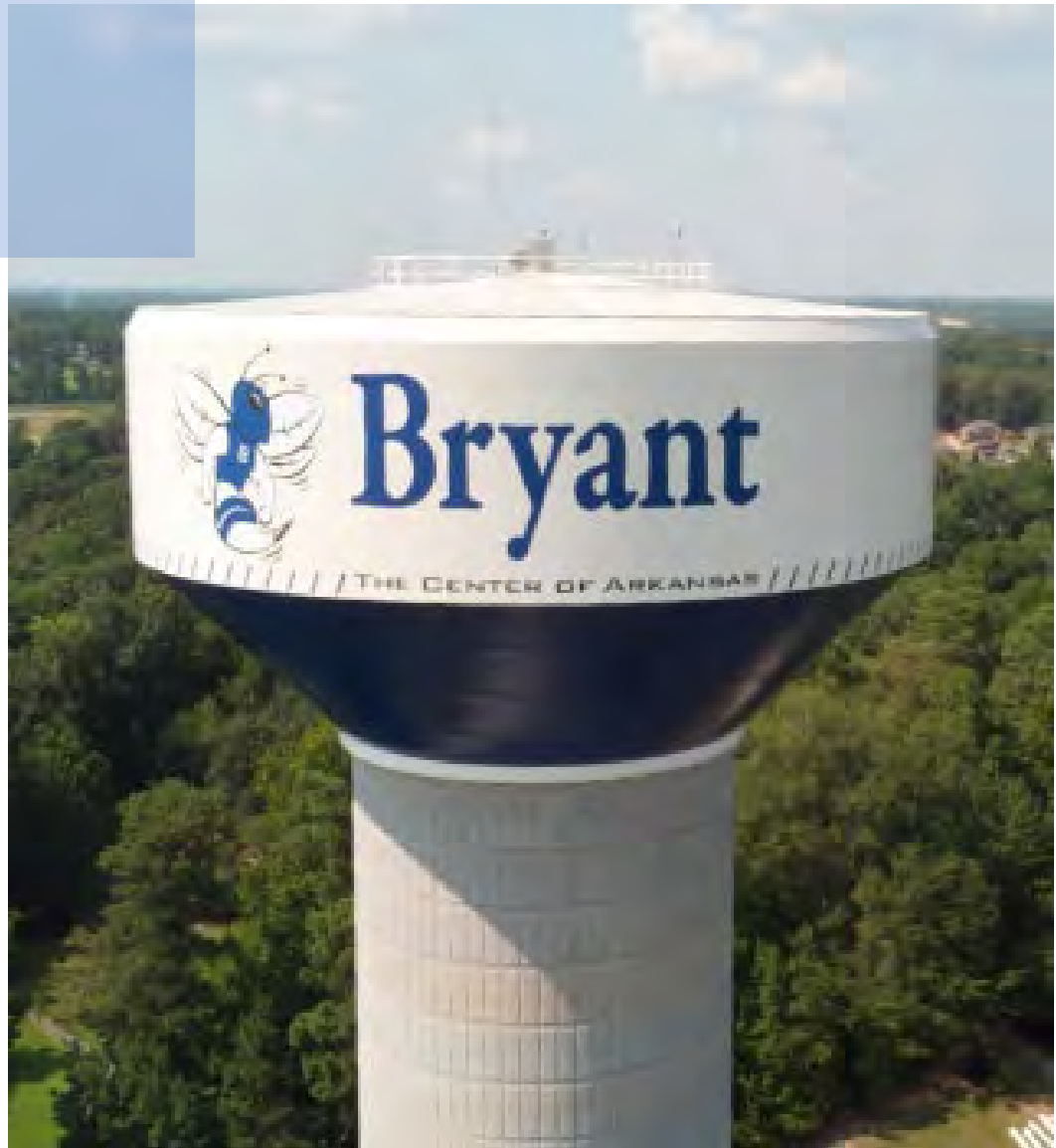
Bryant Water Tower, Hwy 5
